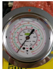
Example of empty (loss of refrigerant)
